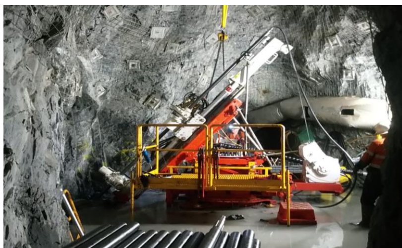
Figure 2. Underground drill rig set up on Level 4 drill cuddy at Dittmer.
