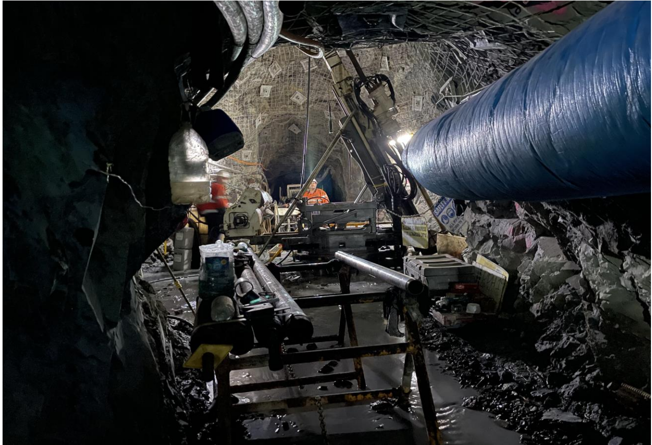
Figure 1 – Drilling of DTDD031 from No. 2 Drill Cuddy, Dittmer Mine.
