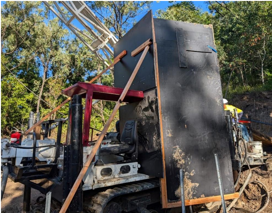
Figure 1 Drill Rig with Noise Barrier Installed Around Engine
