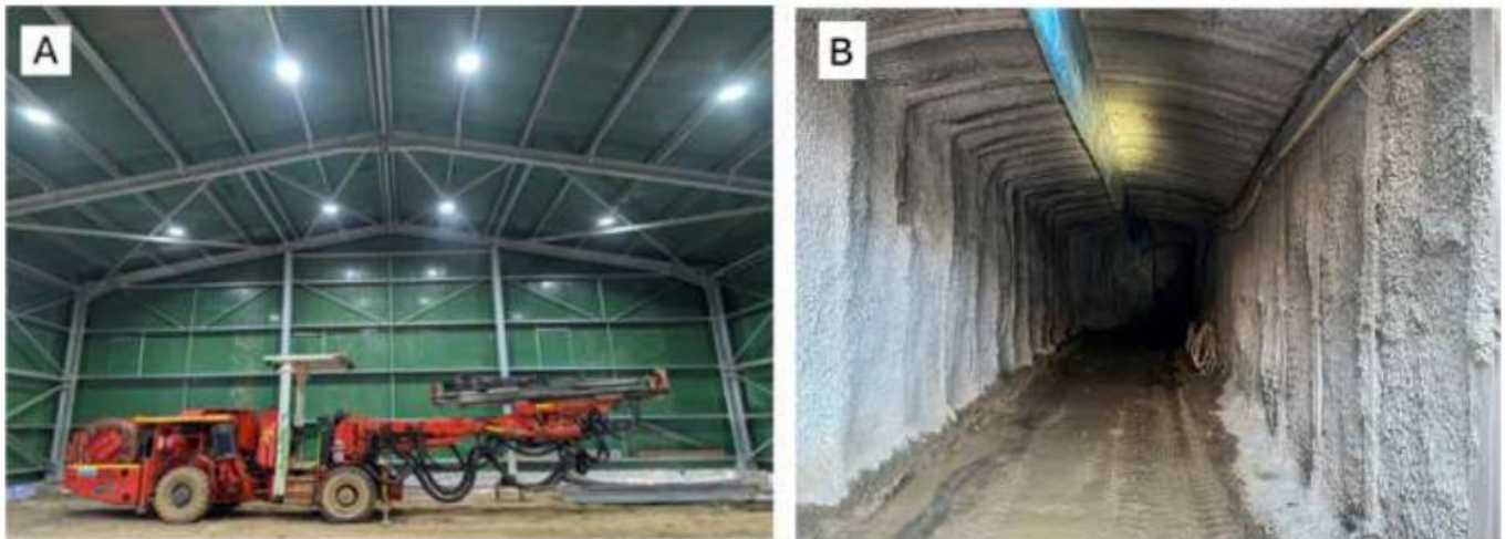
Figure 3 - Photos of the Dittmer mine development. (A) Completed acoustic shed; (B) Portal Shotcreting and Steel Supports.
